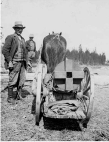
▲ A cart with a roller, designed especially for bike trail construction work. The roller could be attached to the cart wheels and used to compact the bike trail surface.
